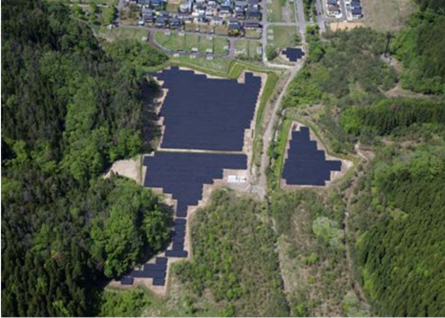
Sendai Project (the whole view)
