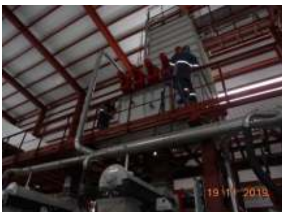
Main production equipment installation
