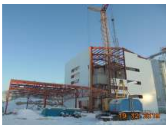
Wood pellet storage/silo construction
