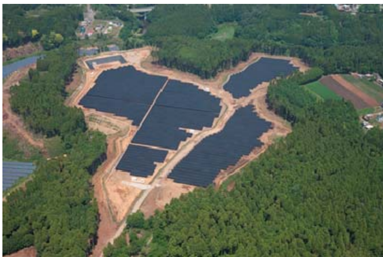
※Sanmu City Shiizaki Solar Power Station
