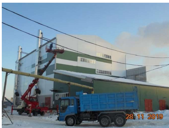
Boiler building construction
