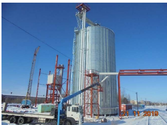
Equipment installation (wood pellet silo/packaging)
