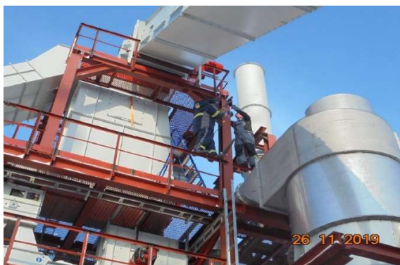
Equipment installation (Hammermill)
