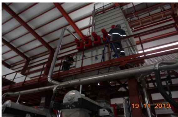
Equipment installation (main production building)
